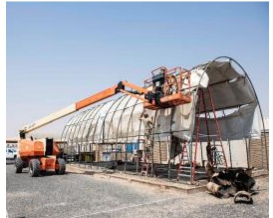
CE TP members using an articulated boom lift to erect an RTC structure.
