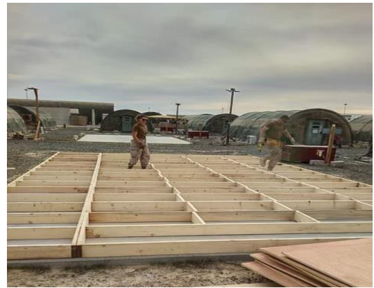
CE TP members constructing a platform to mitigate future flooding concerns.
