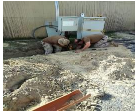
CE TP members installing an electrical cable into a panel.
