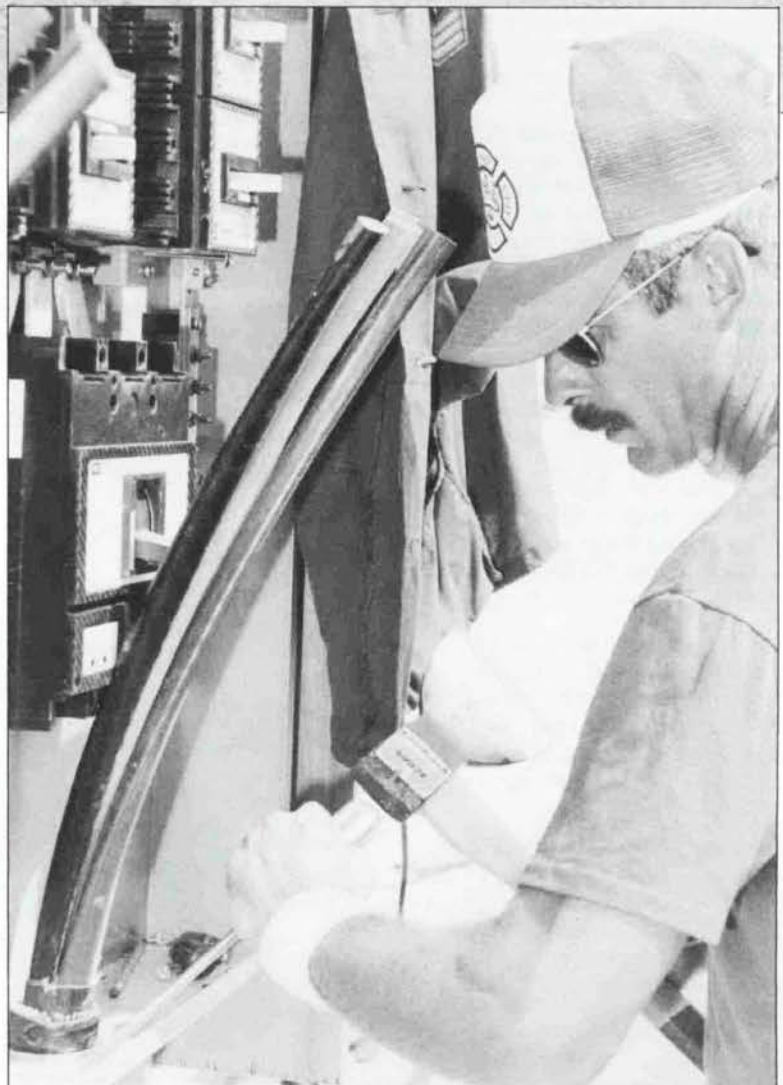
Sgt Bourassa, an electrician from CFB Lahr, is shown installing one of many electrical installations necessary to provide power to all of CD2. Note the size of the cable used due to excessive heat build up in desert environments.
