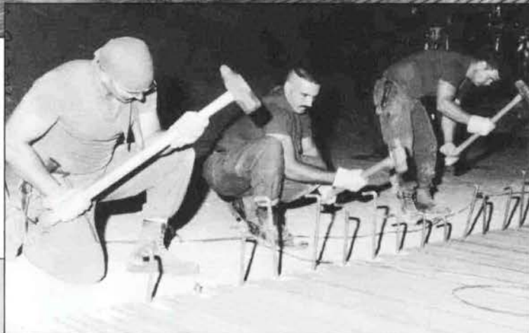
Airfield Engineers worked around the clock for three days to provide much needed ramp space using CL 60 trackway.
